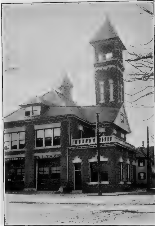
THE PLEASANT STREET FIRE STATION, No. 2.
